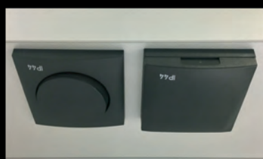
El. socket + switch BERKER is placed outside, on the bottom side of the mirror cabinets TONIC
